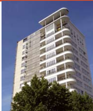
La tour Chaptal, Angers. Photo Atelier Castro Denissof Casti
